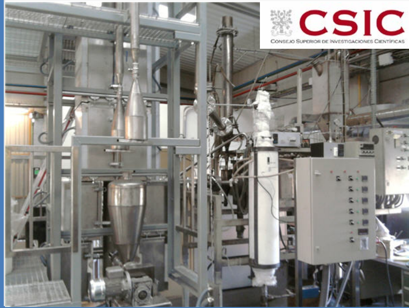
75 kW CSIC-ICB bubbling fluidized bed gasifier
